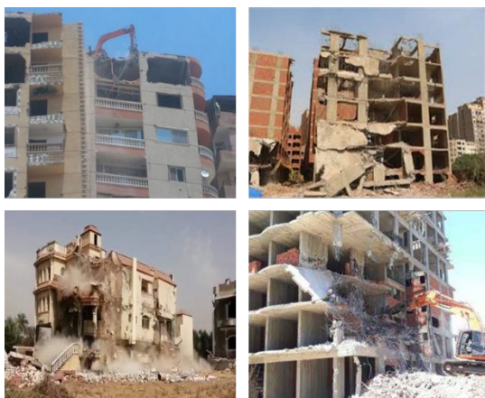
Figure 2. Examples of Demolishing Buildings [25]
