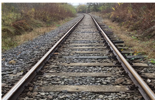
Figure 5. Railway superstructure of the tested section
