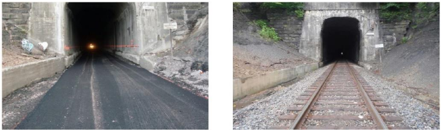
Figure 5. Asphalt layer under ballast [3]
