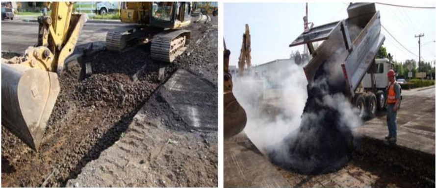
Figure 10. Rail/highway crossing rehabilitation. [1].
