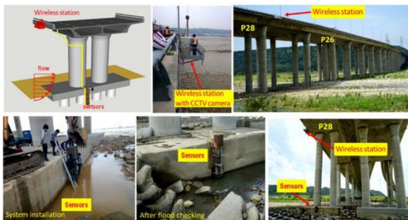
Figure 6. Fixing of the scour observing scheme, sensors, and the wireless station [30].
