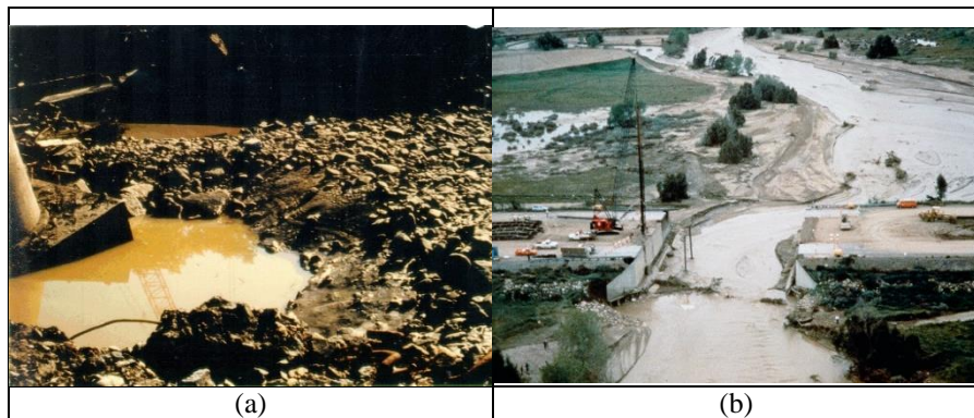
Figure 2. (a) Schoharie Creek Bridge [15] and (b) Arroyo Pasajero [14]
