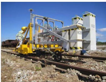
Figure 14. Test equipment of Ground penetrating radar [33]
