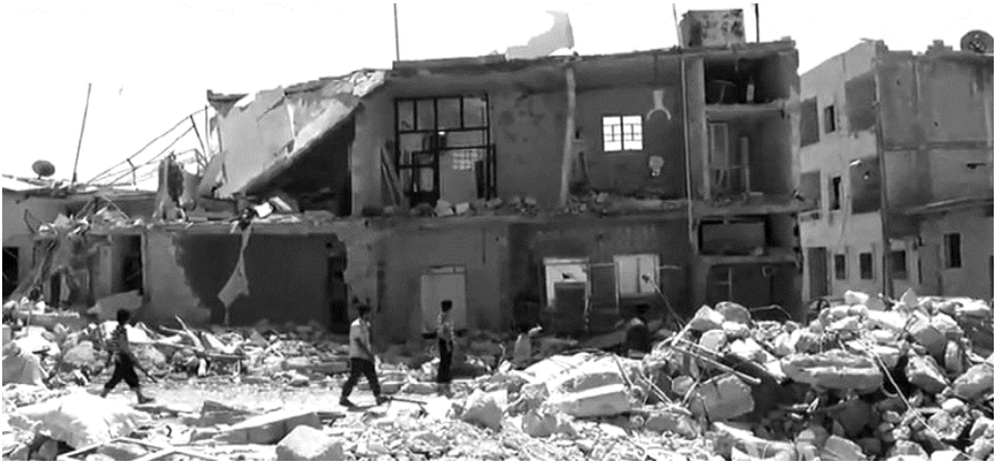
Figure 4. Destroyed place in Syria, with concrete debris [14]
