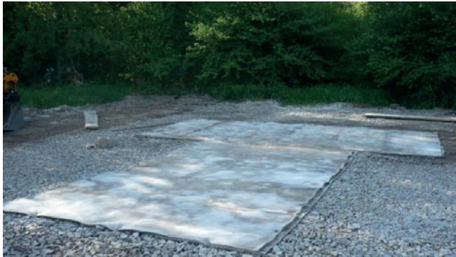
Figure 9. Installing of CC for experimental mobile building foundation [43]
