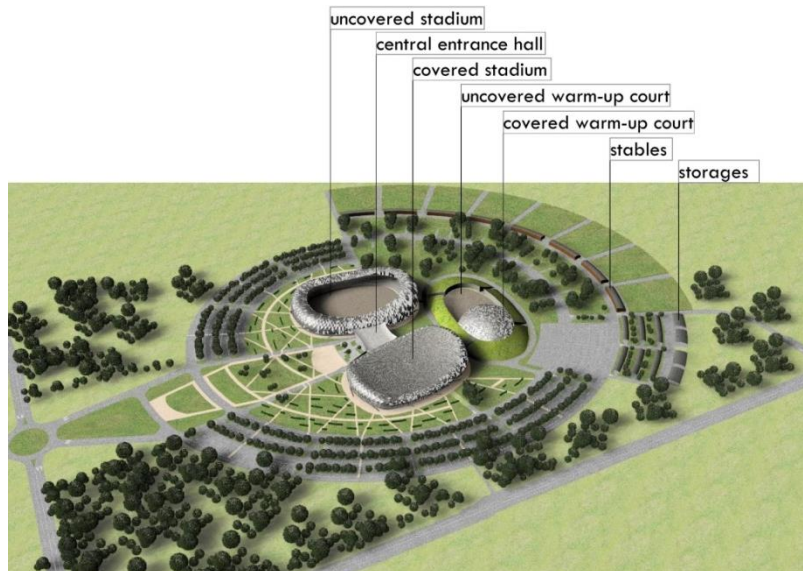
Figure 1. The building complex
